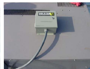
NEMA 4X BOX & HI-INTENSITY UV-C LAMP
